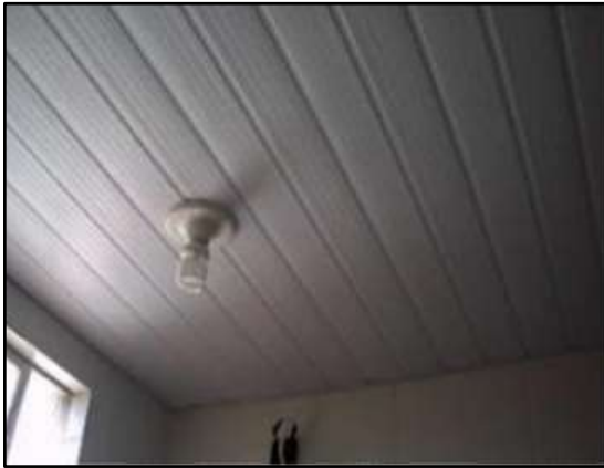
(a) Forro PVC
